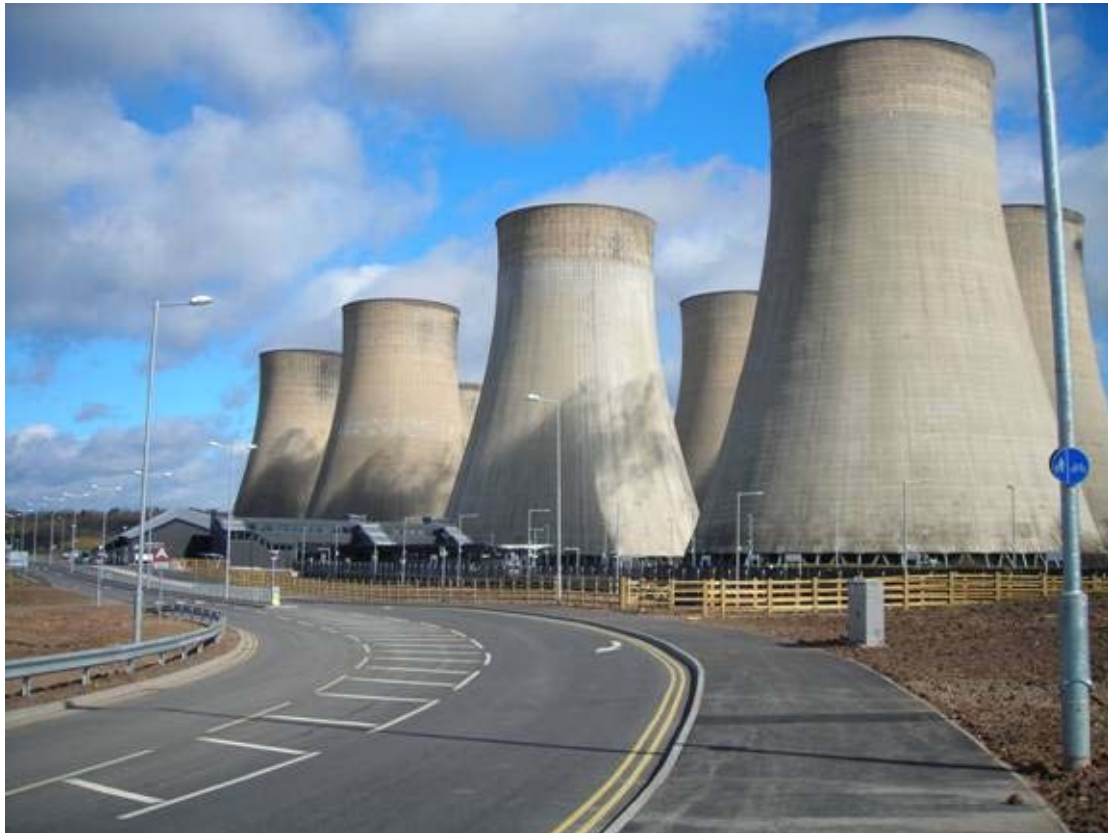
Cooling towers at Ratcliffe on Soar coal fired power station – a hold out for fossile fuels? (see 2 of 2 below)
